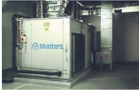
Left: The advanced DryCool™ desiccant system installed at the hospital demonstrates energy savings from cooling and effective reheat. Below: An open DryCool™ unit before complete installation.
